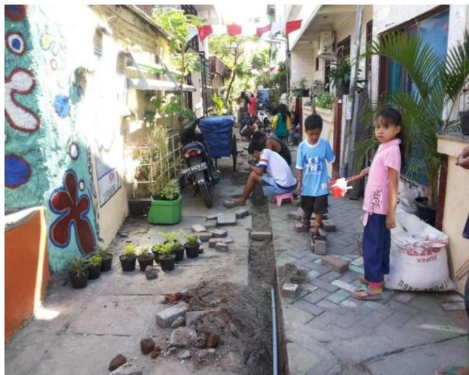
*Figure 7.* Villager's Activity in Rectangular Paving Installation
