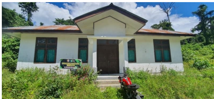
Figure 7. Wartutin district health center that has been built but also has not been functioned due to lack of coordination between the central, provincial government and the local government related to the management of registration at the Ministry of Health (Iha, 2022)
