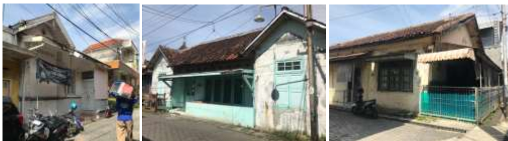
Figure 10. The Fasade Residences (Source: Personal Documentation, 2023)
