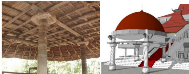
Figure 16. The resemblance between the ume lopo column with the column of Mayor's office building of Kupang City
